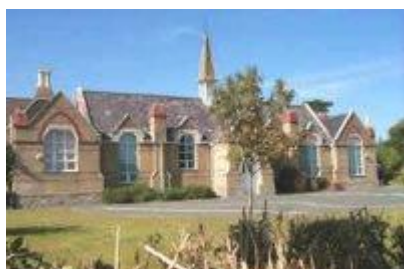
The former Whippingham Primary School building
